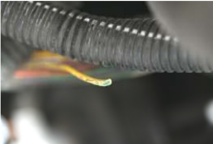
Broken corroded wiring loom causing cutting out
